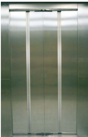
Bus doors – into the car
